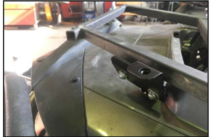
install the housing brackets of relocation box
